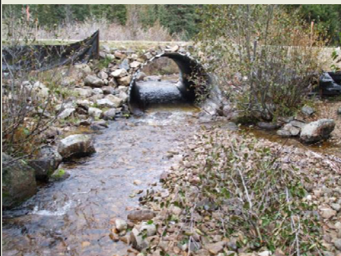
Undersized culvert that contributed sediment to the stream and impeded fish passage
