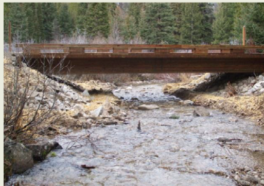
Bridge that was constructed to replace the culvert
